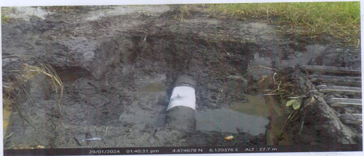
Repaired incident point
